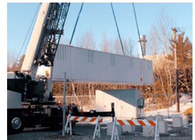
Container Lift of an Agilitas Energy ESS Project
